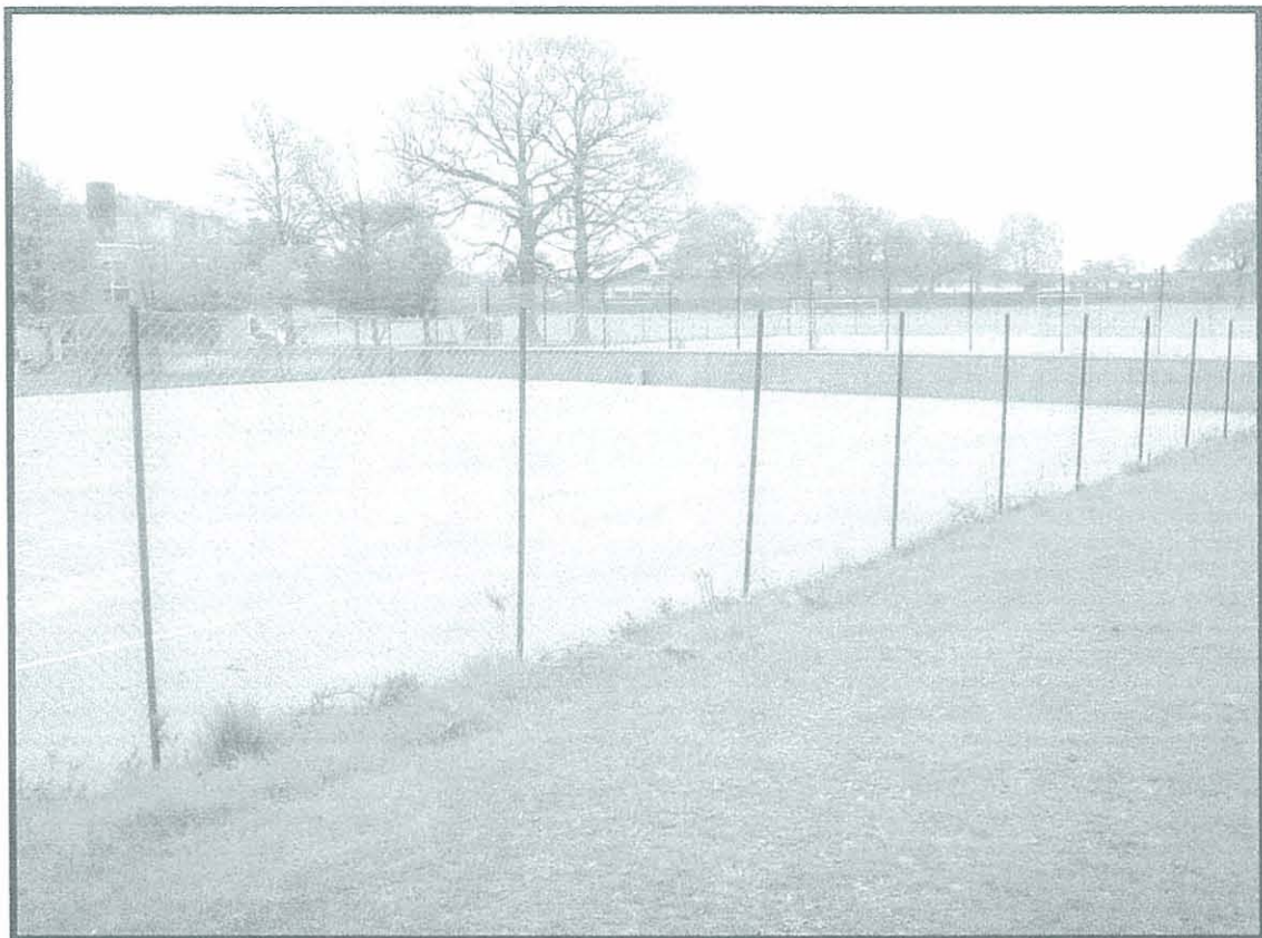
Plate 7 – cuttings created to provide level playing fields and surfaces
